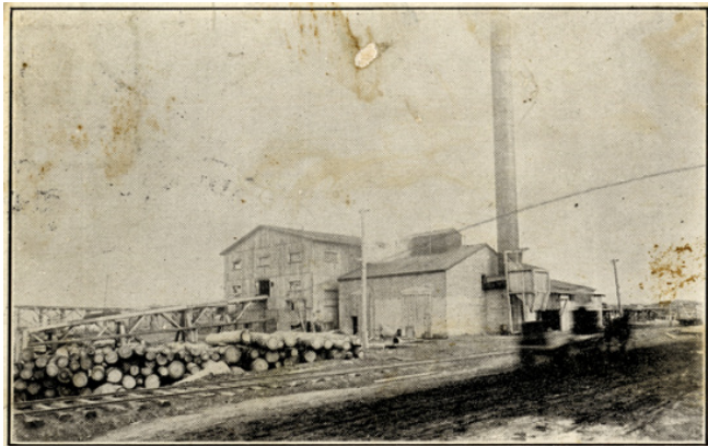
W.H. White and Company Lumber Mill Building.
